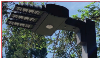
Fig. 1 Typical LED streetlight with topside photocell containing a radio.
